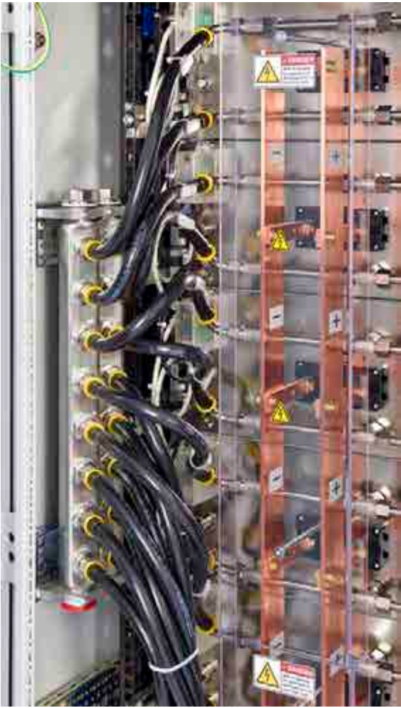
Closeup of the water distribution in a cabinet with eight units and water cooling installed (240 kW system), DC bus
