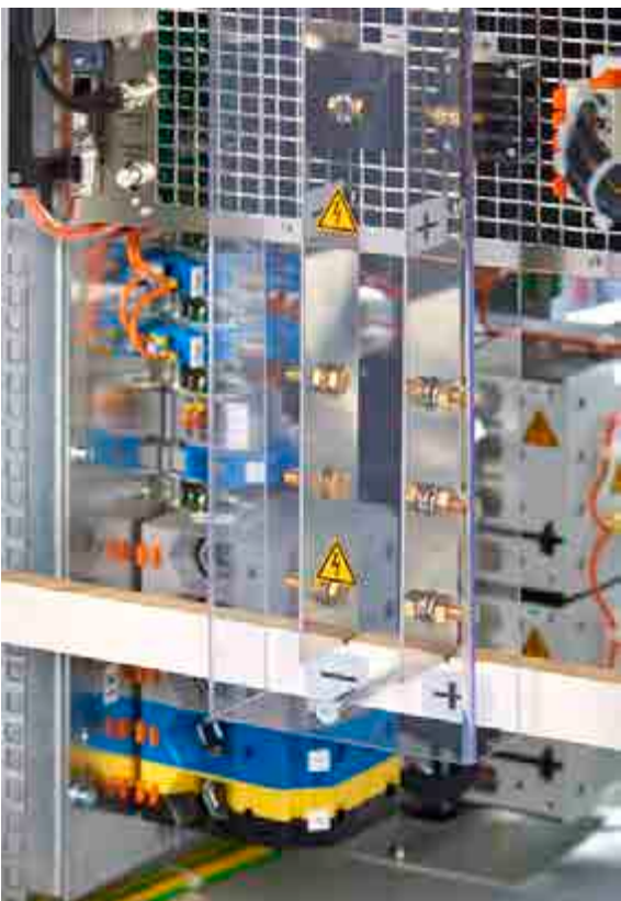
Closeup of the DC bus (24 U cabinet)
