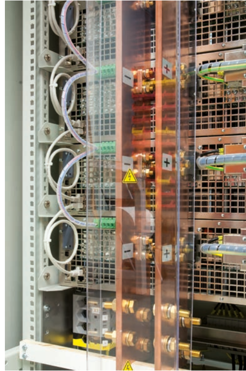
DC bus terminal
